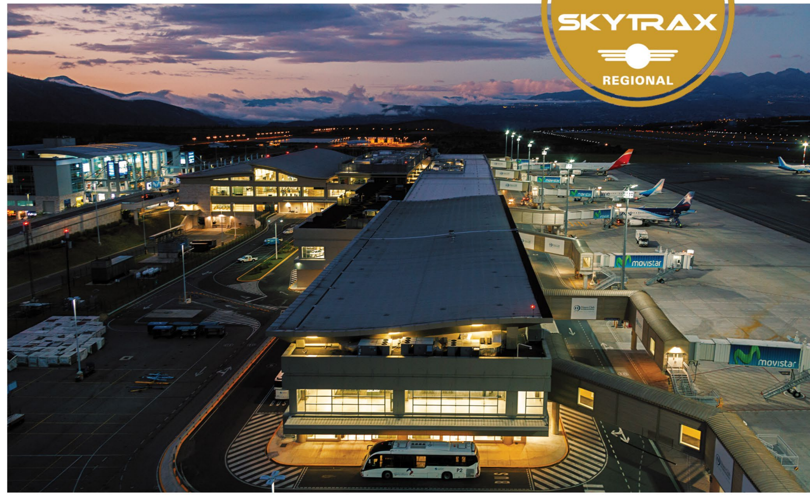
Quito International Airport
